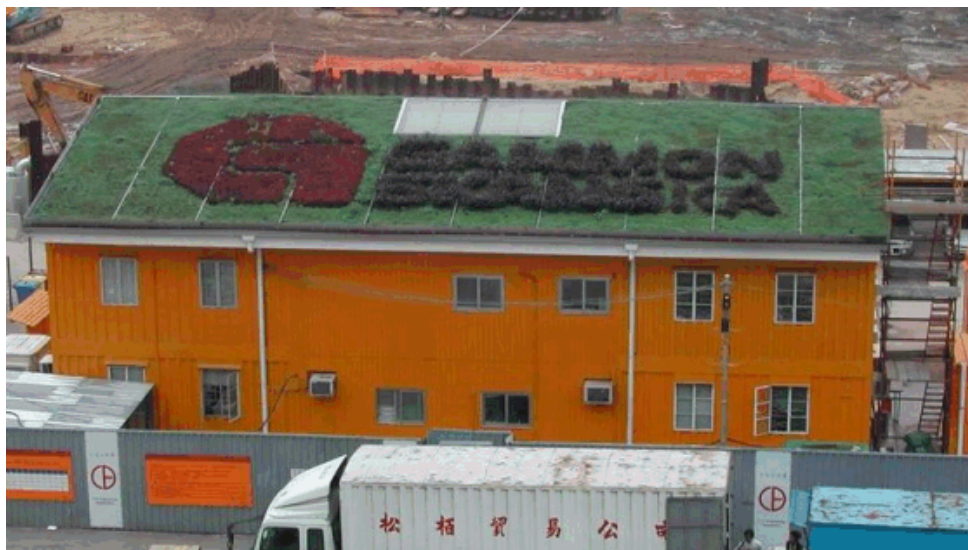
Figure 4. Actual outlook of the green site office
