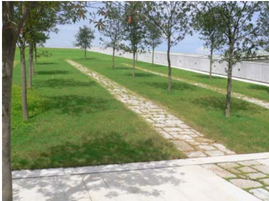
Figure 9. Green roof system at Hong Kong Wetland Park.
