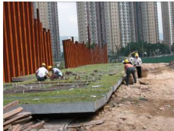
Figure 3. Modular design of the green roof system.
