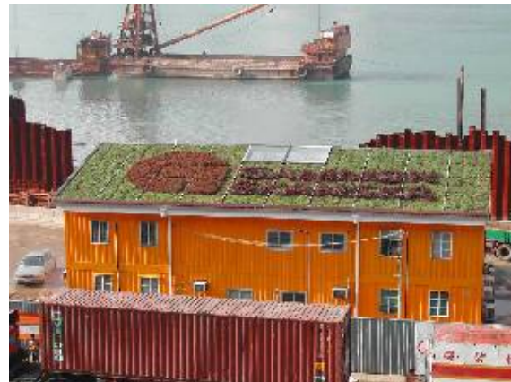
Figure 2. Green roof system installed on a construction site office.
