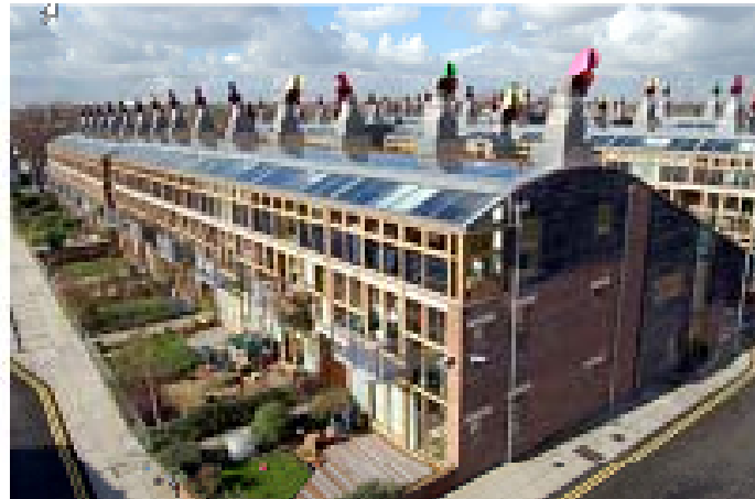
Beddington Zero Energy Development (BedZED), London [2002]
